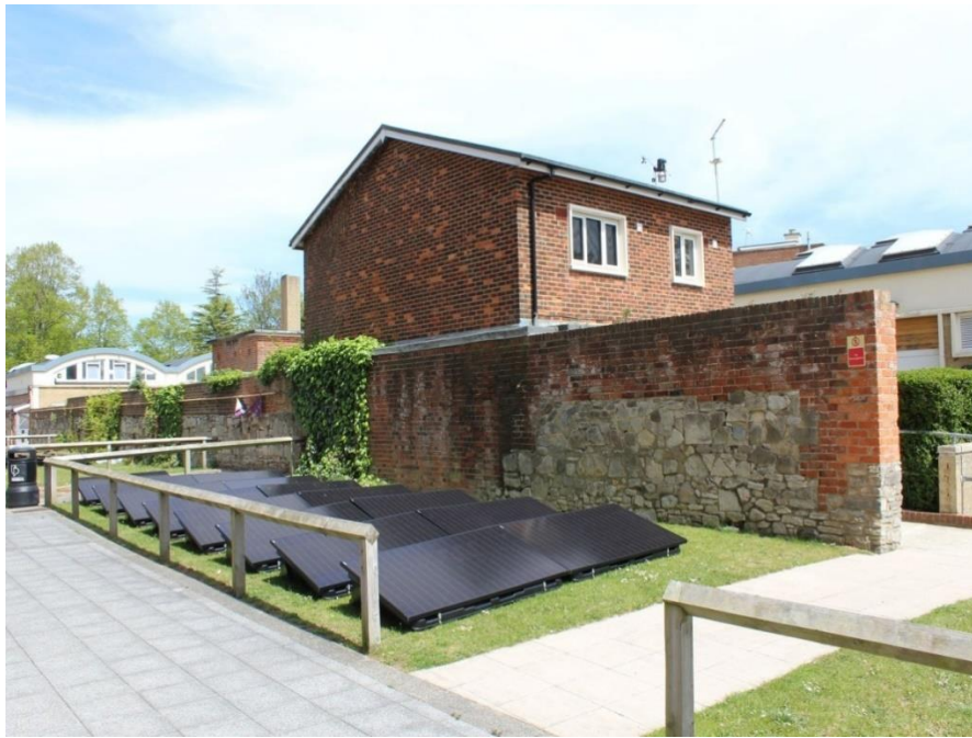
Figure 1: This image shows the installed 5kW photovoltaic solar array on the adjacent lawn by the Port-Eco House, which is shown to the right of the panels.
